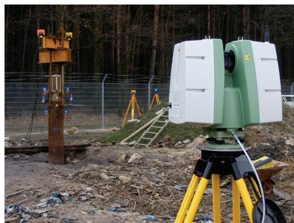
Fig. 1. Application of terrestrial laser scanning to control the vertical displacements during the self-balanced pile capacity testing
